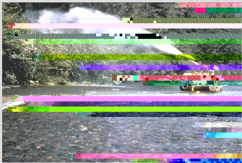
Hydroseeding of a streambank. Source: In Stream Bank Stabilization: Principles, Processes, and Practices (10/99). By the Federal Interagency Stream Restoration Working Group.
